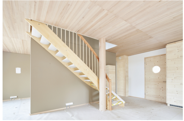
TS3 technology allows for a column-and-slab construction method. The TS3 joints remain visible in this project.
