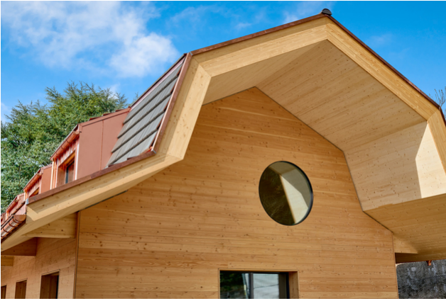
From the outside and inside: Timber remains visible and gives the building a pleasant atmosphere.
