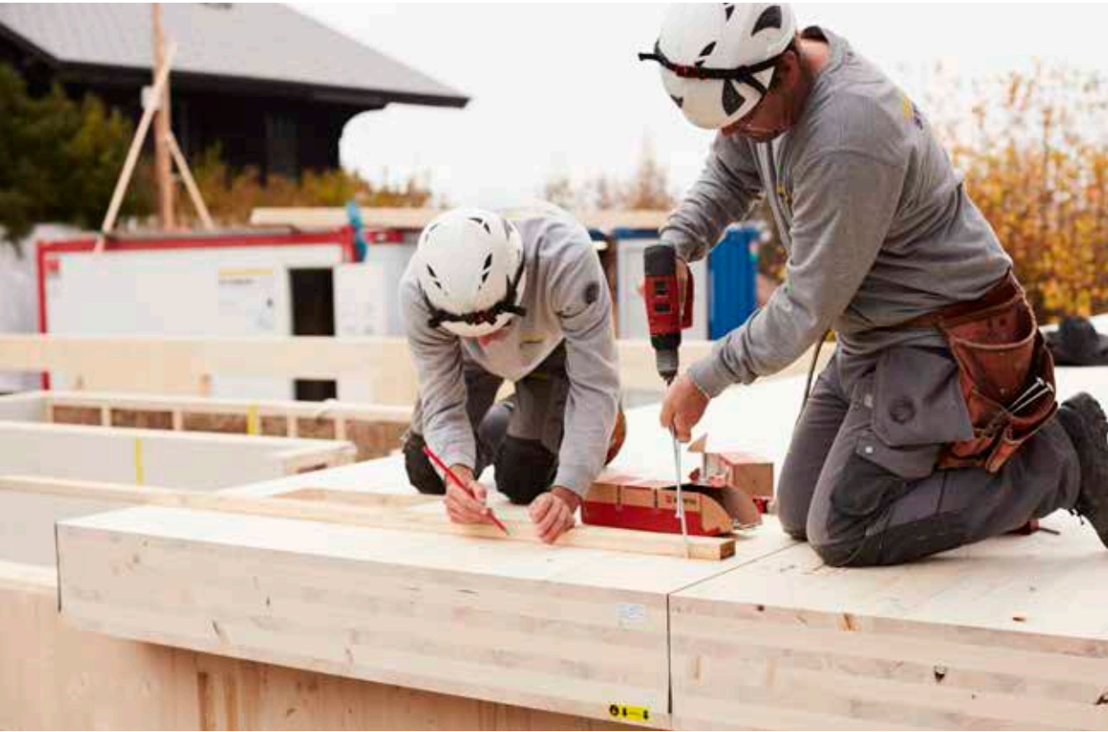
Assembly of the CLT base plate covering the timber basement.
