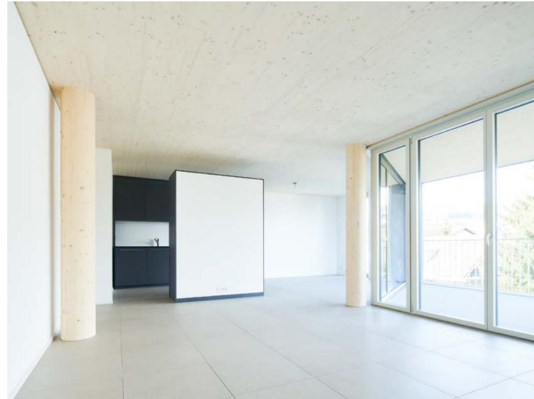
The core technologies are the column heads and the end-to-end liquid jointing of the wooden components. Both are the result of multiple research projects with the Bern University of Applied Sciences and the Federal Institute of Technology in Zurich. The cost of this system is comparable to that of a reinforced concrete ceiling.
