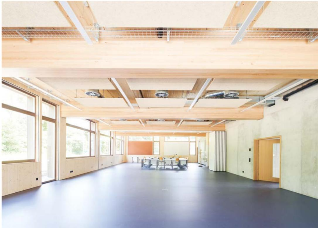
Large beams interfere with the installation of building services.
