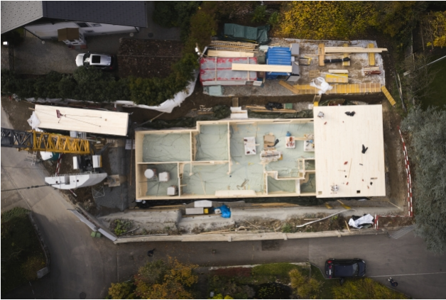
What seemed impossible for a long time is now a reality: Thun is home to the first apartment building with a basement made entirely of timber.
