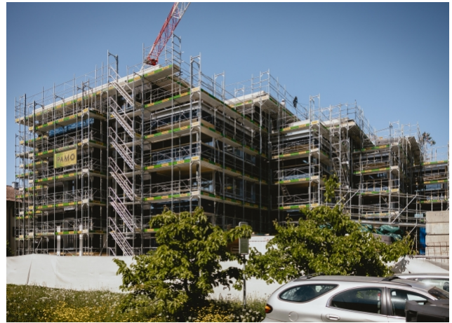
Block of flats Luegisland - Construction phase 2
