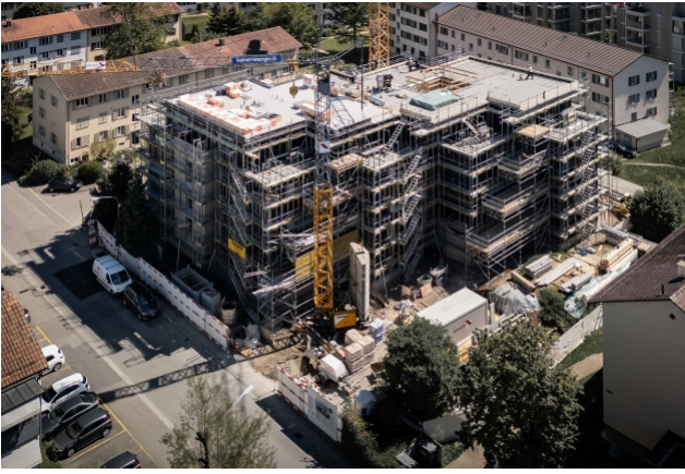
Block of flats Luegisland - Construction phase 1
