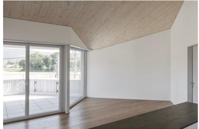
In the case of the apartment buildings on the lower right bank of Lake Zurich, the advantages of TS3 technology and timber construction are both noticeable and visible: the construction method allows flexible room division and timber ceilings that run from the inside to the outside without complex cantilever connections.
