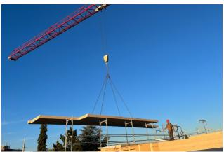
The existing apartment building from the 1980s on Bahnhofstrasse in Busswil was extended with an annex and raised with an attic floor. With the TS3 system, the extension was able to fully utilise the building regulations without losing room height due to beams.
