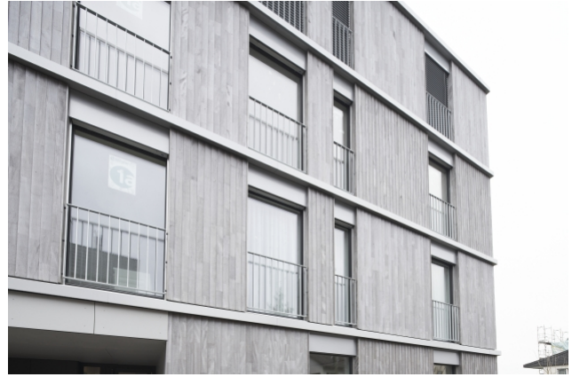
The building was once planned in concrete. TS3 technology made the switch to wood construction easy.
