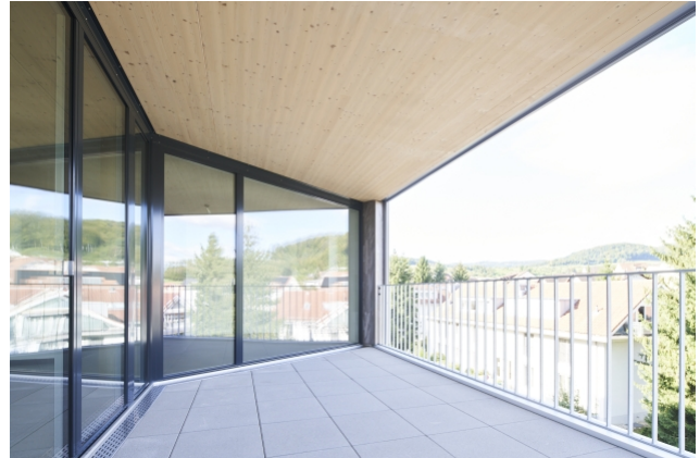
Thermal bridges made simple. CLT ceiling simply runs through from the apartment to the loggia.
