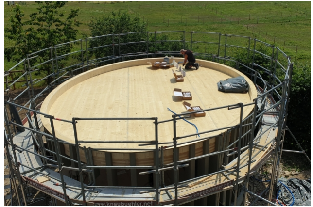
Assembly work on the roof of the pavilion
