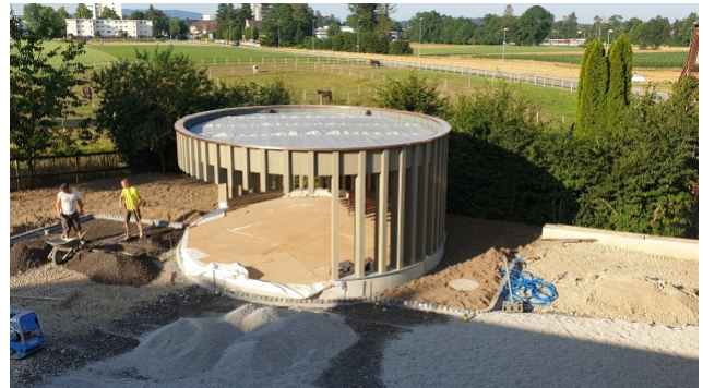
Construction work around the pavilion
