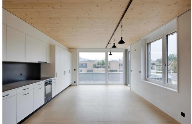
The new replacement building at Wehntalerstrasse 52 in Zurich-Unterstrass has eight apartments of different sizes. The ecological aspects as well as the longevity are of great importance for the Generationenhaus W52. The slabs of all storeys are made of TS3.
