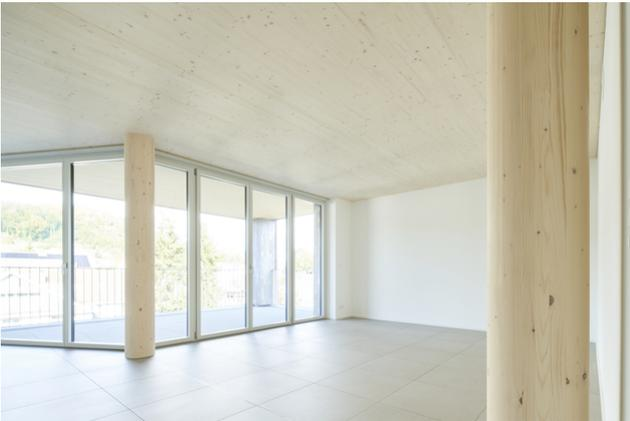
Thanks to the load-bearing support, the walls are not load-bearing and can be easily moved.
