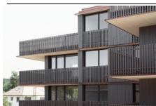
Apartment houses Unterhub, Zollikerberg
