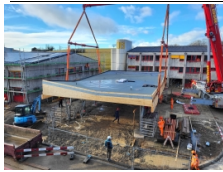
Barracks roofing, Chamblon , Chamblon
