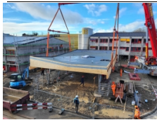
Barracks roofing, Chamblon , Chamblon
