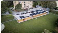
Roofing technical building swimming pool, Martigny , Martigny
