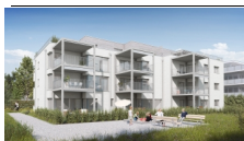
Extension Bahnhofstrasse, Busswil , Busswil
