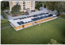
Roofing technical building swimming pool, Martigny , Martigny
