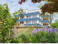
Residential block Zollikerstrasse 211, Zürich , Zürich
