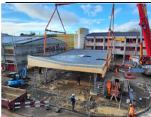
Barracks roofing, Chamblon , Chamblon
