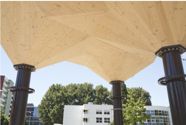
The wooden shells are supported by eight steel columns
