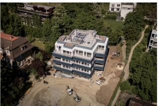
The new building is based on a pure TS3 skeleton construction with point-supported flat slabs – completely without beams. The ceilings, made of continuous CLT panels, connect the interior and exterior spaces both visually and structurally. Balconies and living spaces merge seamlessly – a key quality of the TS3 system. The ribbon windows emphasise the openness and provide light, views and airiness – supported by the filigree supporting structure made of the TS3 cast resin composite system.
