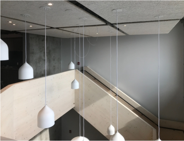
The first staircase with TS3 technology
