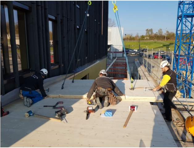
Mounting the CLT panels
