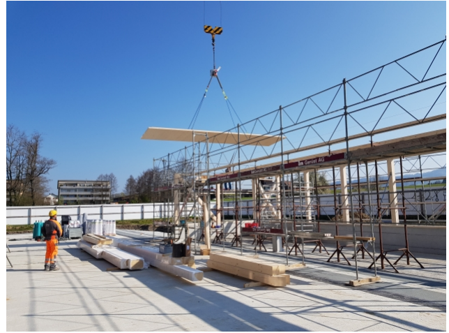
Mounting the CLT panels
